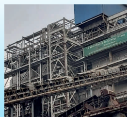
Waste to Energy Plant
